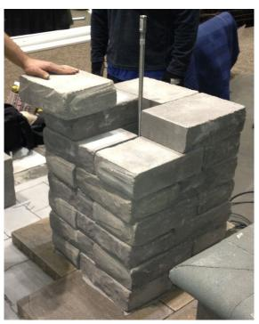
Install the Cambridge Column Kit following the instructions from Cambridge Paving Stones. If using a cap stone, drill a 5/8 or larger hole into the center and slide over the threaded rod.
