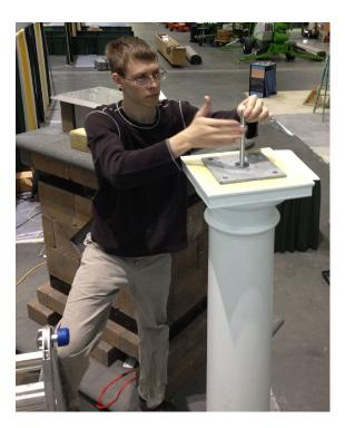
Slide column over threaded rod and attach final rod section. Slide Cap and Base onto column before attaching top plate. **Tightly** secure top plate using provided nut and washer to complete column assembly.
