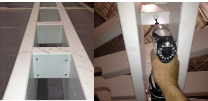
Align rafters with the spacers between the Beam Assembly. Secure by putting the long self tapping wood screws through the bottom of spacer, and into the rafter above.
