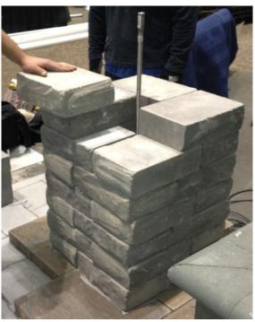
Install the Cambridge Column Kit following the instructions from Cambridge Paving Stones. If using a cap stone, drill a 5/8 or larger hole into the center and slide over the threaded rod.
