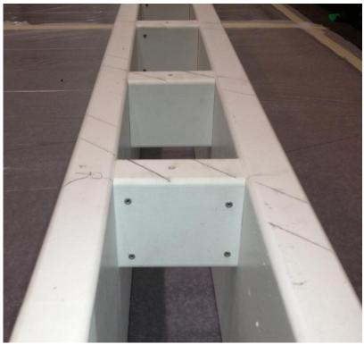
Align rafters with the spacers between the Beam Assembly.
