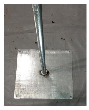
Cut two of the 6 foot sections of threaded rod into 4 three foot sections, you will need at least 2 inches of rod protruding above the cap on the paver pedestal.
