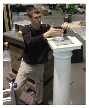
Slide column over threaded rod and attach final rod section. Slide Cap and Base onto column before attaching 10 inch aluminum top plate. Check that column is plumb then **Tightly** secure top plate using provided nut and washer to complete column assembly.
