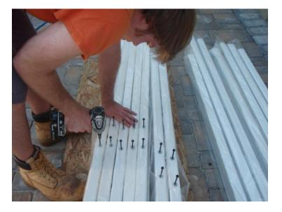
Predrill holes in the top of the rafters on the ground first then start the long gold screws into the holes.
