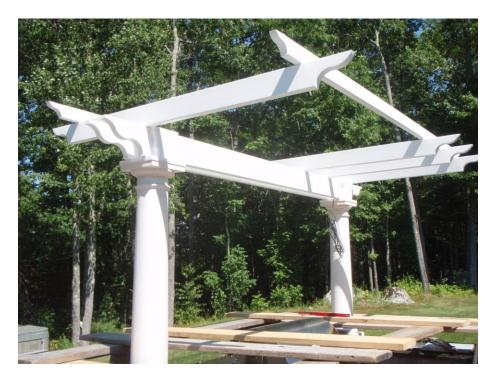
Set then and level the leftmost and rightmost rafters first. Then set the backmost and frontmost purlin. Double check level on both rafters and purlins. Begin installing the remaining rafters and then install the remaining purlins.
