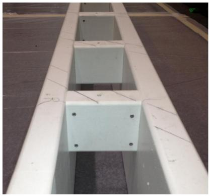
Align rafters with the spacers between the Beam Assembly. Secure by putting 9 inch wood screw through pre drilled hole in **bottom** of spacer, and into the rafter above.
