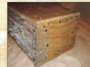
Scratch-coat of mortar applied.
