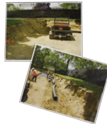
Photos of future retaining wall site
